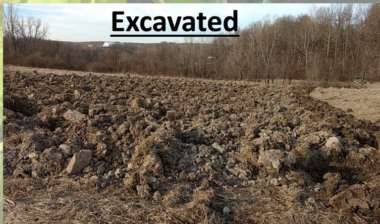
Fig. 4—Here you can see the result of the excavation method. Developed by David Polster, this method involves a track hoe digging a 3-4 ft deep hole, then emptying the bucket half next to the hole and half back inside the hole. A tree is planted in the side of the resulting pile.
