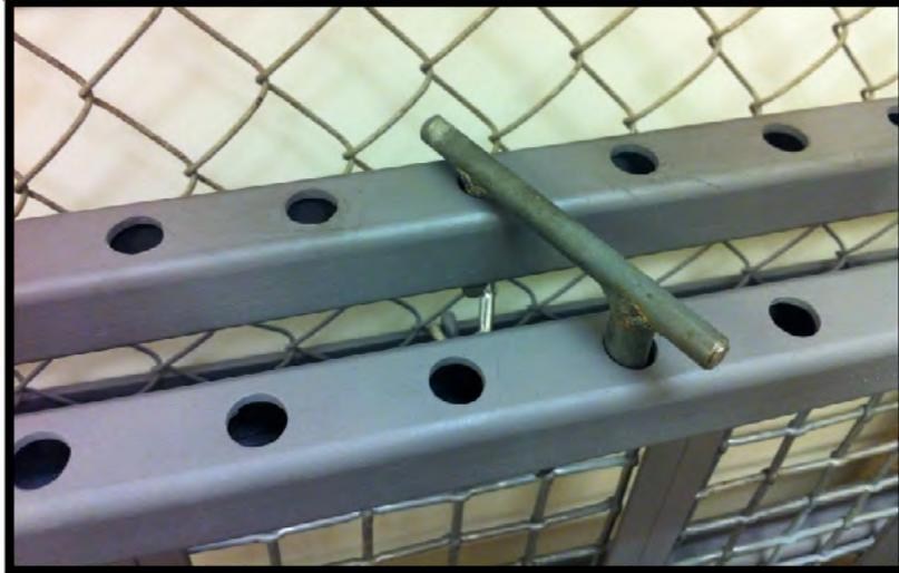
**Figure 13** - A top view of the two "C" bars pinned together when closed so the hogs cannot move the chute from the other side of the enclosure.
