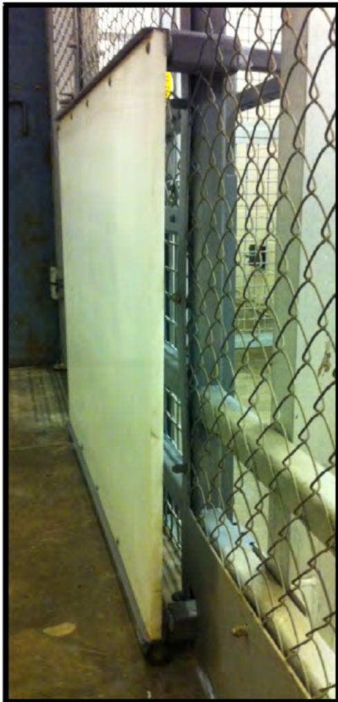
**Figure 7** - This is a side view of the chute closed with the panel pulled against the wall.
