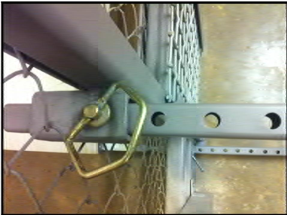
**Figure 10** - The top view of the chute shows the holes in the "C" bars on the top and bottom that are pinned to position the wall at different widths.
